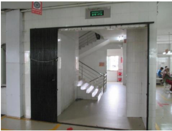
Before: Collapsible Gate
