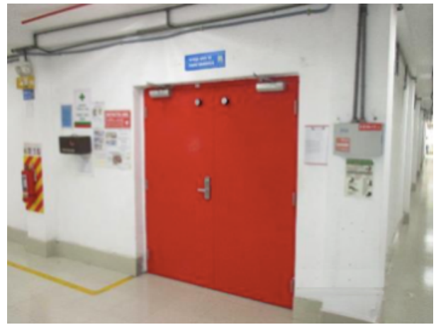
After: Fire Door Installed
