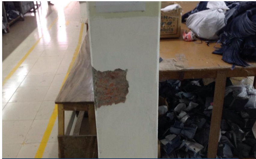
Tested ground floor column – brick aggregate
