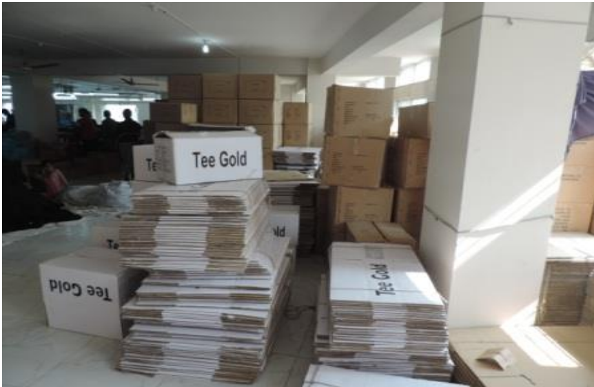
Uncontrolled loading on level 3
