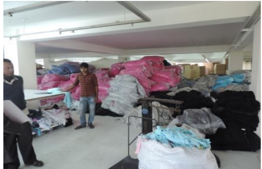
Uncontrolled loading on roof
