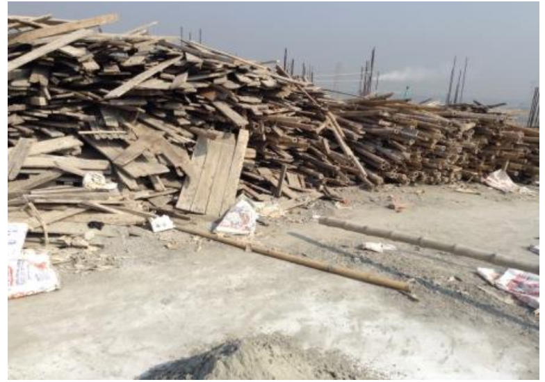
Uncontrolled loading on roof
