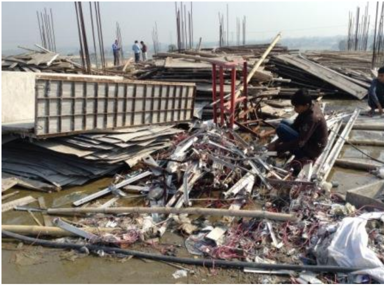
Uncontrolled loading on roof
